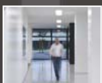
Corridor and staircase lighting Page 20
